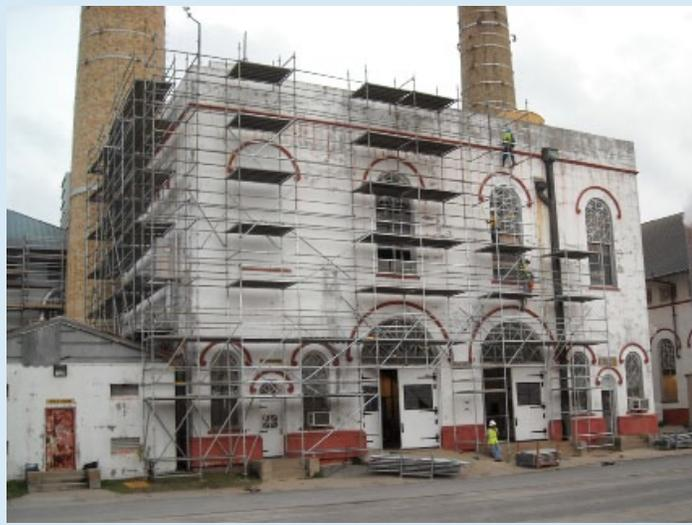
*These storm proofing measures have been completed with the Power Plant Complex. These measures included, but not limited to, water intrusion protection, roof and wall reinforcement, strengthening of louvers, doors, shutters and ventilation systems and miscellaneous electrical and mechanical equipment storm proofing measures.*
