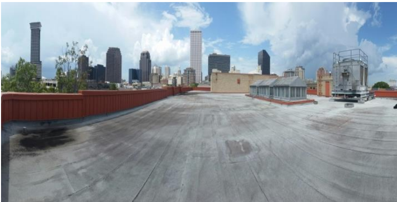
Existing roof at 625 St. Joseph St.
