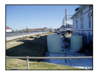
Figure 37. Temporary Sodium Hypochlorite System
