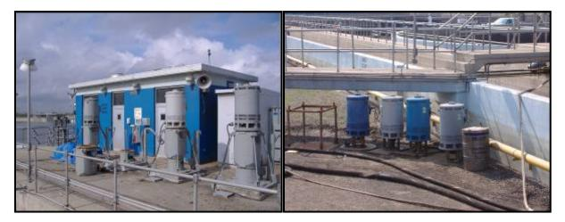
Figure 20. Solids Transfer Pumps
