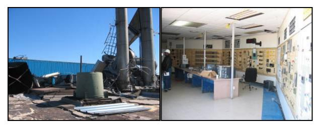
Figure 21. Damaged Incinerator Stack & Control Room
