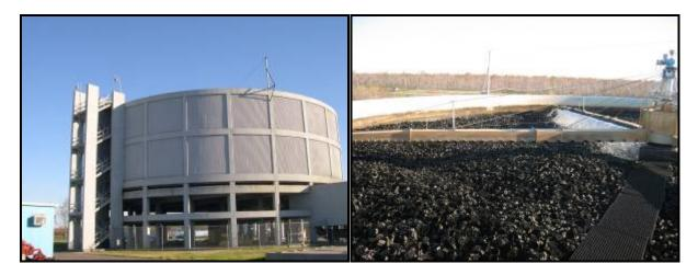
Figure 29. Trickling Filter & Packing Media
