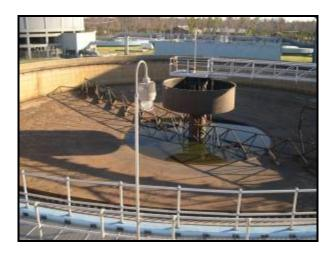
Figure 30. Jammed Rake in Primary Clarifier
