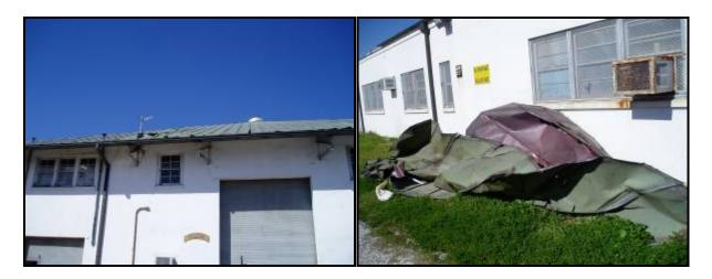
Figure 36. Roof Damage to Maintenance Building
