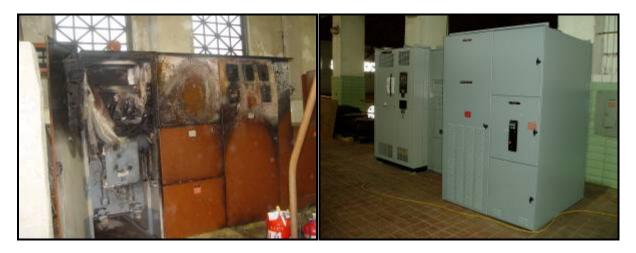
Figure 9. Damaged/New Turbine No. 3 Switch Gear
