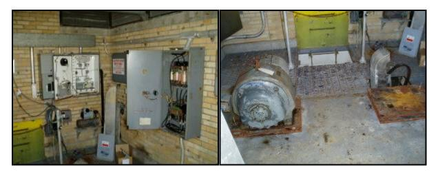
Figure 31. Damaged Electrical Components
