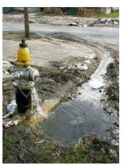
Figure 38. Water Distribution System Leaks
