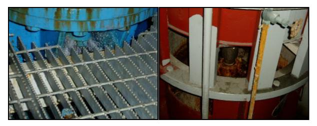
Figure 15. Water Leaks – Panola & Claiborne Pumping Stations
