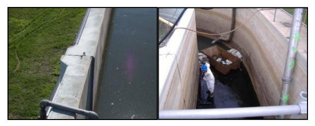
Figure 17. Wall Separation in Effluent Channel
