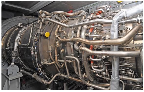
burn oil, gas or a mixture of the two. The gas turbine, at present, operates on fuel oil. Two fuel storage tanks, with a total capacity of one million gallons of oil, provide reserve fuel supplies.
