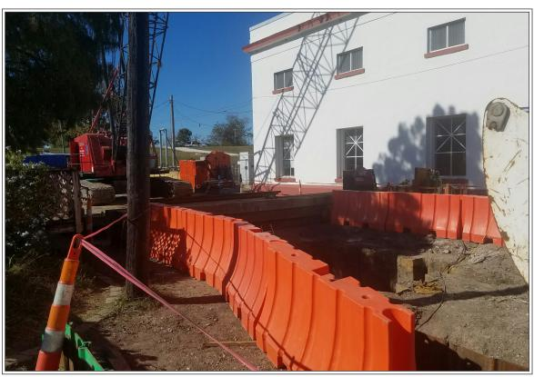
The S&WB Oak Street Pumping Station Rehabilitation is part of the Hazard Mitigation Grant Program. The existing station has 4 pumps that pump water from the river to the S&WB Carrollton Water Plant to be treated. This construction will remove three pumps and replace them with brand new motors and pumps, along with new piping and auxiliaries. Completion is expected in 2019. However, high river levels can cause a delay in the construction outside the
