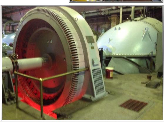
The Drainage system of today dates back to the turn of the century. The New Orleans Drainage Commission was established in 1896 and merged with the Sewerage and Water Board. This is a photo of drainage pump C at Drainage Pumping Station No. 6. The station was built in 1899 on the 17th Street Canal. Pump C was commissioned in the 1920's to add to the station's drainage pumping capacity. Today, as with pump C, many of the drainage pumps at the station have been refurbished, rebuilt or upgraded.
