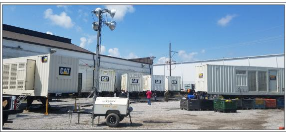
Generators were put in place at various facility sites to provide an uninterrupted power source to critical operations. They were designed to increase and insure reliability in the event of a commercial power interruption.
