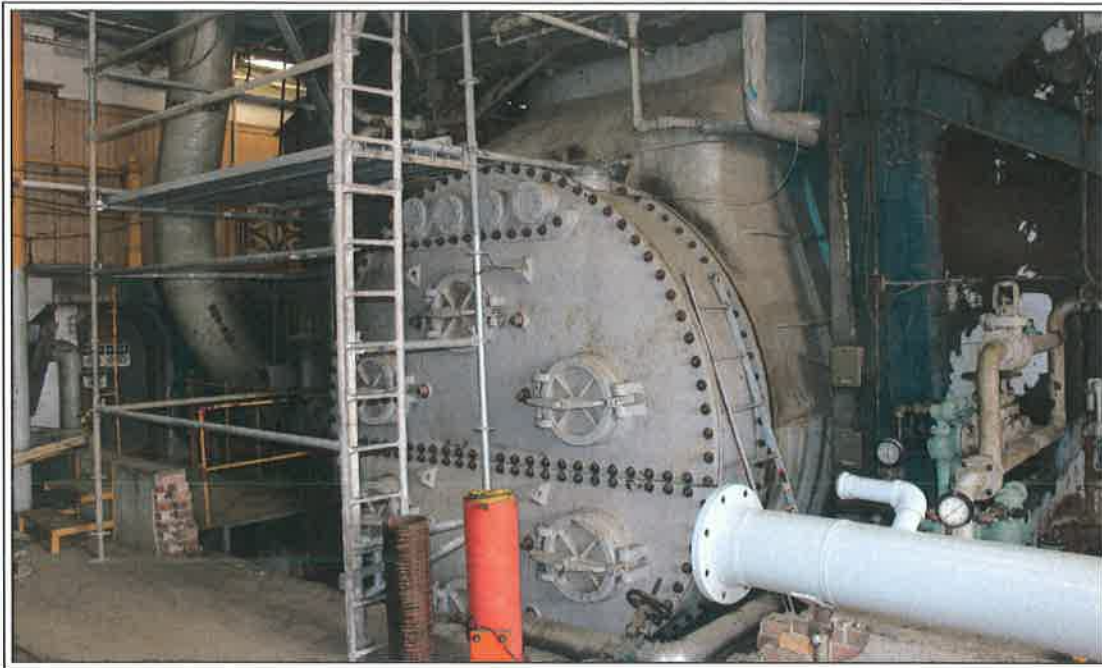
The board's 25 cycle Power Generation System, located at the Carrollton Water Plant, provides power for portions of the Water Purification Plant, two large vertical sewer units at the main central business district sewage pumping station and powers approximately 60 percent of the system's drainage pumps. The benefit of the board's own power generation is that the feeders to the multiple pump stations are underground and during storms when commercial power lines are down the system is still up and running. Shown is a component of the power plant which is the Turbine 4. Funding from FEMA for repairs to the power house has included the boiler, repairs to Turbine 4, A and B steam pumps, replacement of high lift turbine equipment and replacement of the boiler pre-heater. Under FEMA public assistance, the board has a FEMA 404 Hazard Mitigation Grant for the Retrofit and Hardening of the power houses equipment and building. The combined amount of funds received is $232 million.
