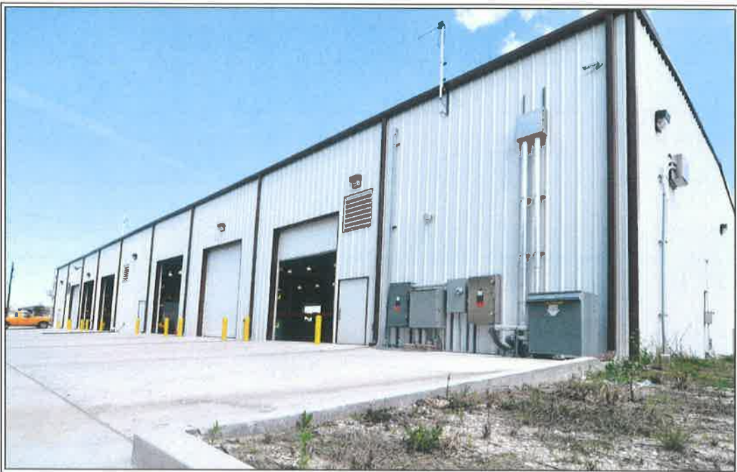
The vehicle and equipment repair and service garages at Central Yard are being repaired and constructed. These facilities are critical to operations. Thus, FEMA funded a facility to serve as an interim location to service light and large vehicles and heavy equipment. This new facility is a temporary location while Garages I and II repairs and construction is completed. It houses personnel and equipment needed to service the vehicle fleet and equipment. It is called a site relocation facility. The FEMA funding for the project was $1.8 million. Upon completion, the new garage will be the home of the body shop. Besides the garages, Central Yard is the service facility of the board. The site, also, includes support services, networks, meter reading, environmental affairs and the warehouse.
