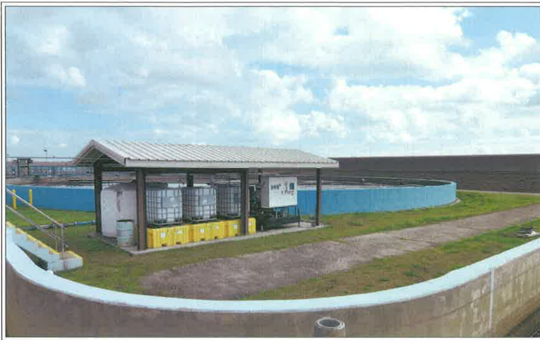
The ferrator system at the East Bank Sewage Treatment Plant is designed to fully disinfect the effluent prior to discharge to the wetlands, with no residual effects or by-products. This new technology is being used in a pilot trial with the wetlands. In the foreground is the current effluent channel where all of the water that is currently treated is disinfected prior to discharge to the Mississippi River. Behind the Ferrator is a Final Clarifier that will be the source of water used in the first phase of the Wetlands Assimilation project, a partnership with Orleans and St. Bernard Parishes.
