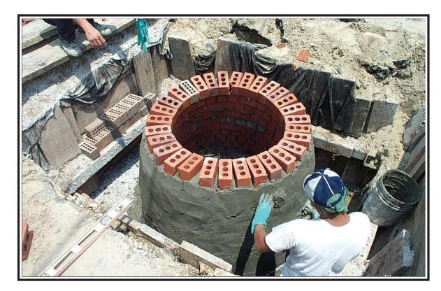
A major element of the Board's Sewer System Evaluation and Rehabilitation Program (SSERP) is the replacement of damaged, leaking or sinking manholes. Since 1998, approximately 4,800 sewer manholes have been repaired or replaced. Above, a manhole is under construction, and below, the completed structure is ready to be sealed into a new section of roadway.
