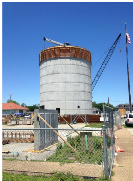
Water Tower Construction
