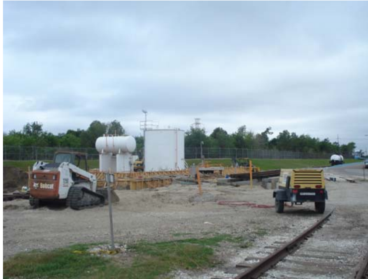
Figure 3. Site of New Generator Building
