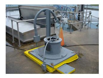
Figure 6. RAS Pump Out for Repair
