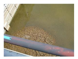
Figure 2. Sediment buildup in Chlorine Contact Basin C5/C6
