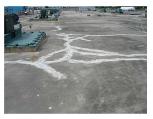
Figure 7. Repaired Cracks in Deck
