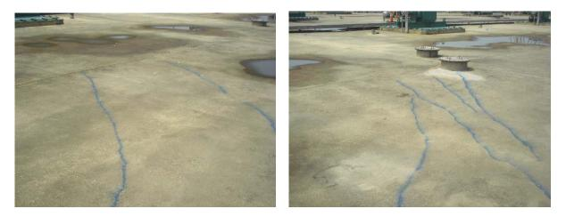
Figure 7. Cracks in Deck
