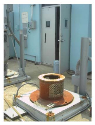
Figure 8. RAS Pump Out for Repair
